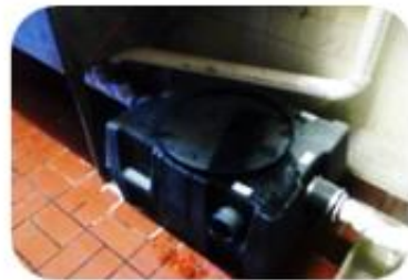
High Capacity Hydro-mechanical Grease Interceptor
